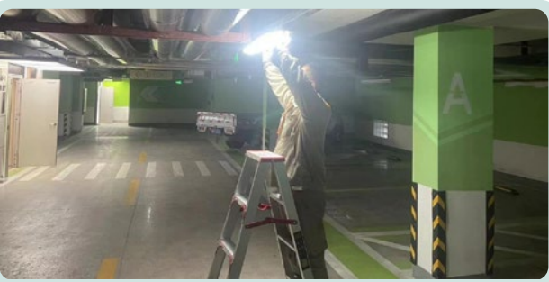
Replacement of constant lamps to LED radar dual-brightness lamp
